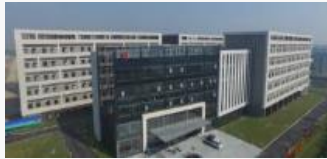
Ningbo Laboratory services 2.56 million ft 2
