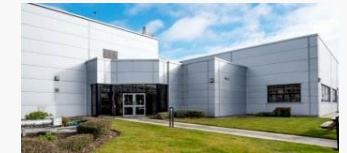
Cramlington Commercial API Mfg. 60,000 ft 2 (production area)
