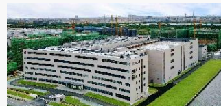
Ningbo Campus II Biologics CDMO 350,000 ft 2
